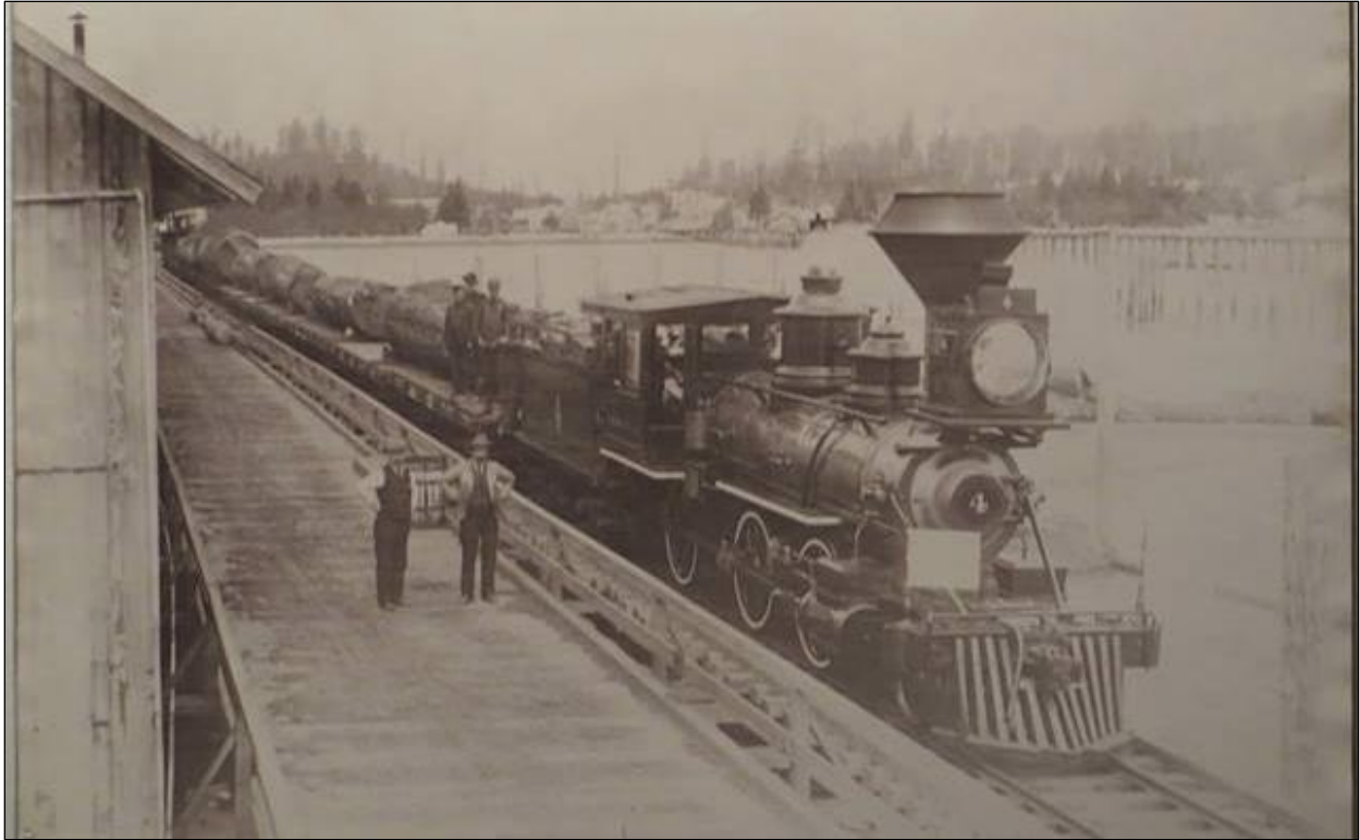
Figure 11. Overview of the Ilwaco Railway and Navigation Company terminus at the Ilwaco Wharf. Photo courtesy of Oregon Historical Society.
