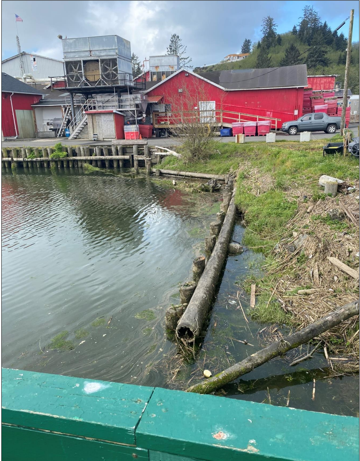
Figure 5. Overview of the shoreline/slope between the East Bulkhead and the West Pier. View facing west.
