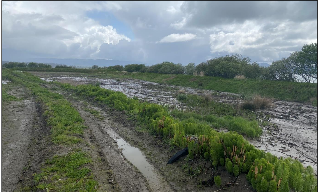
Figure 7. Overview on top of dredge placement at southeastern end of study area. View facing east.
