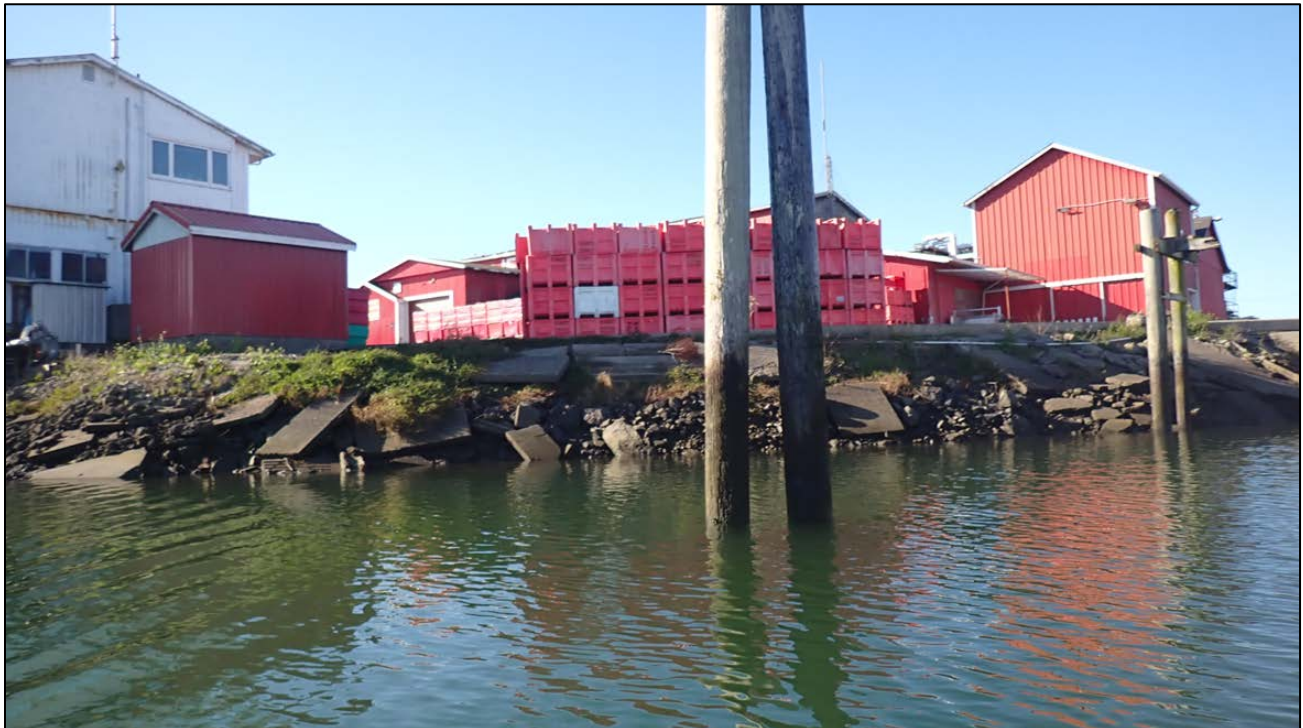
Figure 3. Rip Rap Shoreline to the South of the Bulkhead Wall
