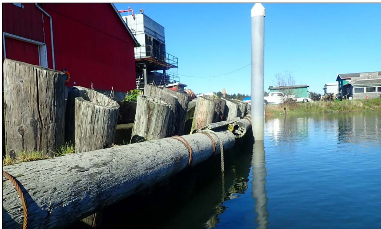
Figure 1. Damaged Bulkhead Wall
