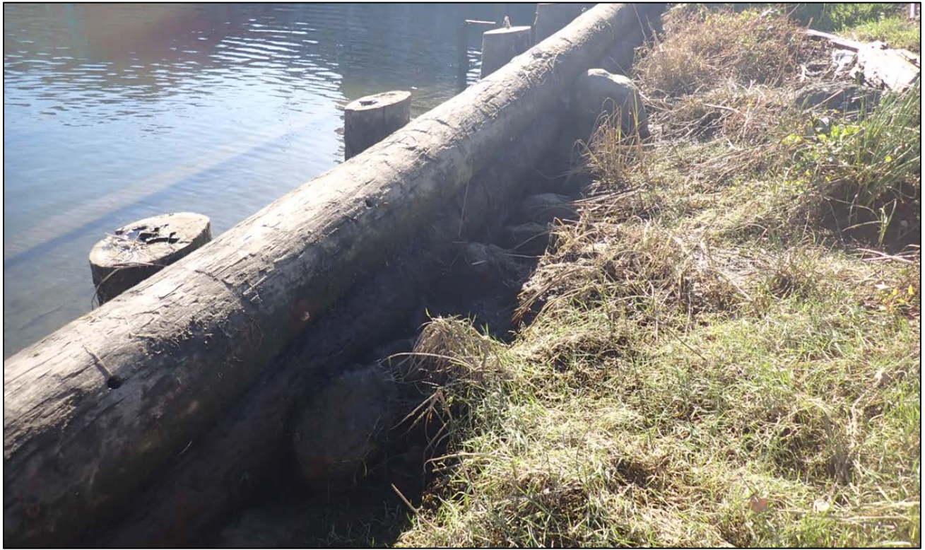
Figure 4. Retaining Wall to the North of the Bulkhead
