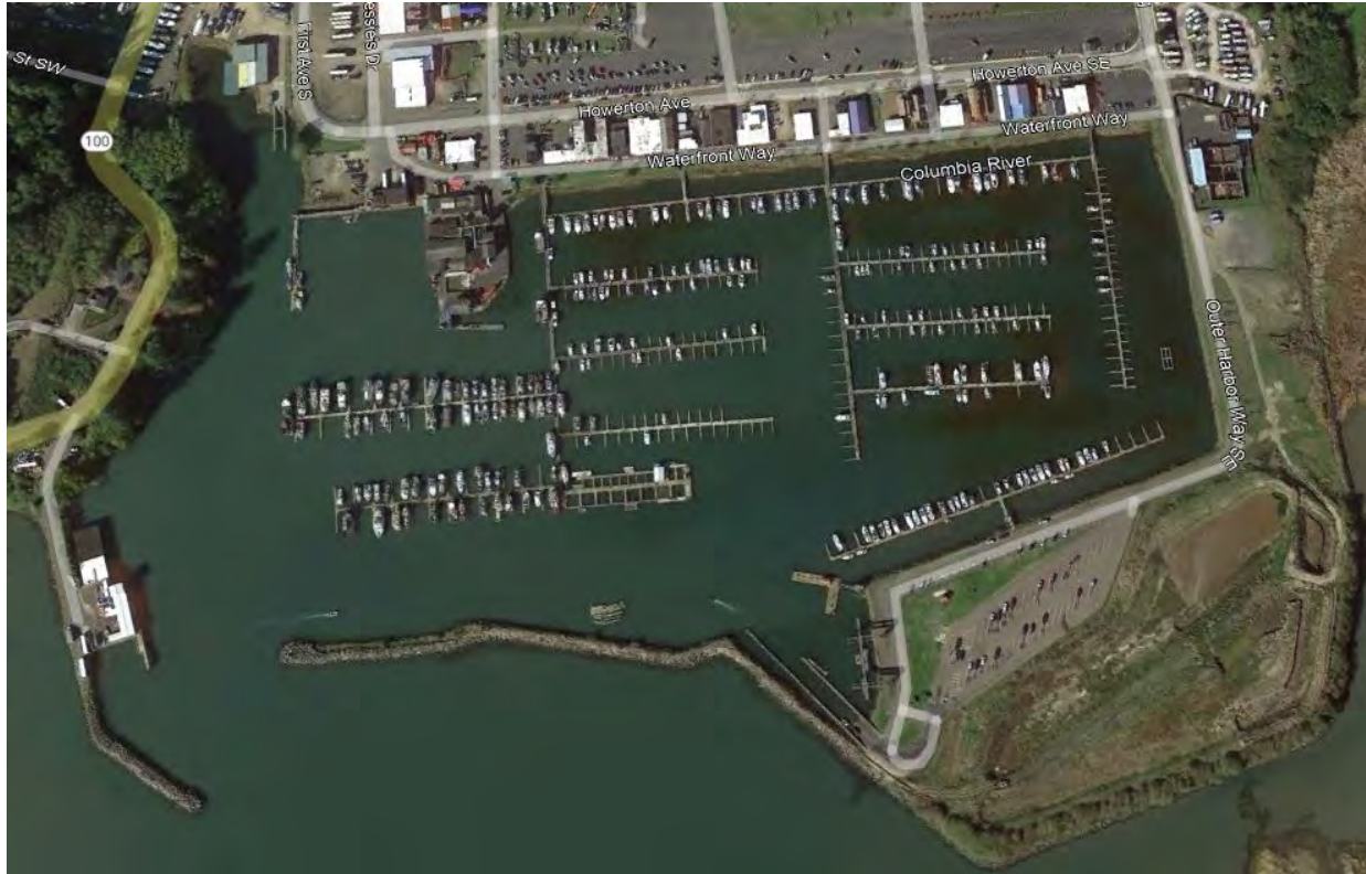
Figure 2. East bulkhead resilience project action area
